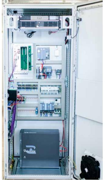
In most applications the WiC is a bypass or an "add-on" system to the existing combustion control system. It may also be integrated from project start up. The WiC usually comes in a cabinet of 600D x 800W x 2000H mm (24D x 31W x 79H inch) and is placed in the DCS room.
